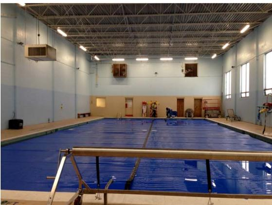
**Figure 3: Pool Blanket after Installation**
