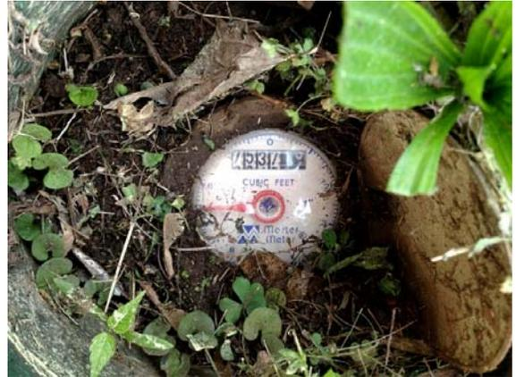
**Figure 4: Irrigation System Submeter**
