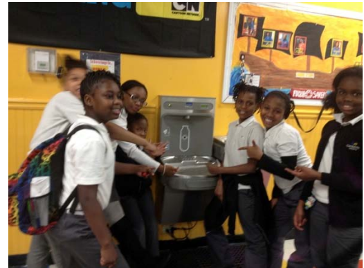
Figure 5: New Drinking Fountain with Bottle Fill Station
