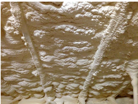
Figure 3: New R-20 Spray Foam Insulation in Attic
