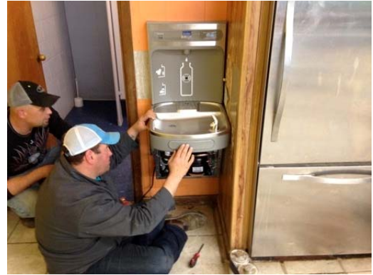
Figure 4: Installing the Drinking Fountain
