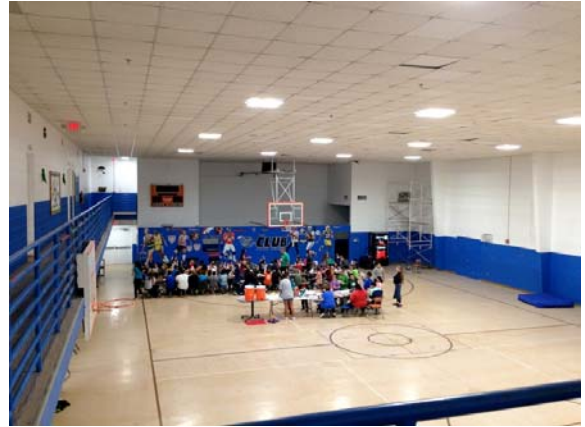
Figure 4: New LED Lighting & Controls Throughout
