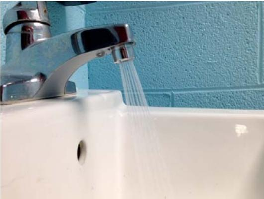
Figure 2: New 0.5-GPM Aerators
