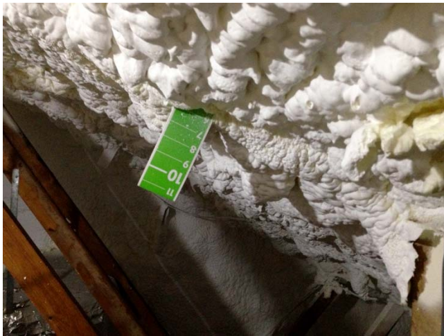
Figure 2: New R20 Spray Foam Insulation
