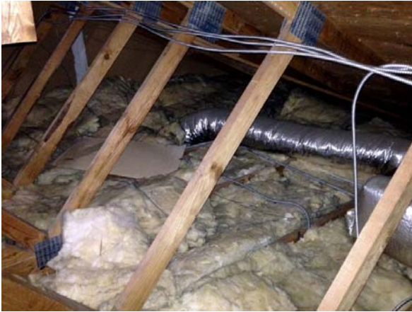
Figure 1: Original Insulation over Suspended Ceiling
